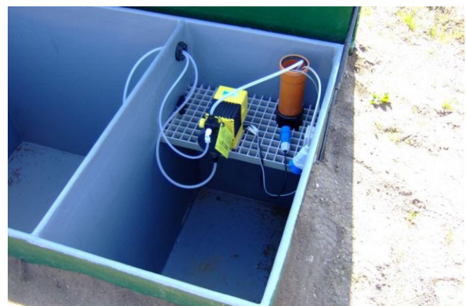
Figure 3. The facility in Silkeborg. On the left hand picture the lid of the container for aluminum dosing is seen. On the right hand picture, the dosing pump and space for a pallet containing the aluminum is shown.
